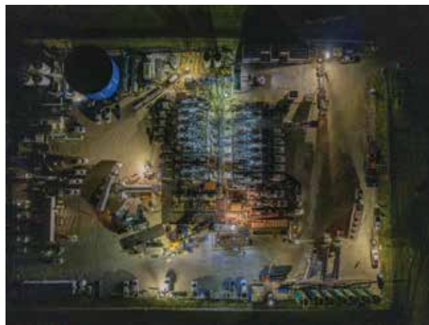
Universal Pressure Pumping
